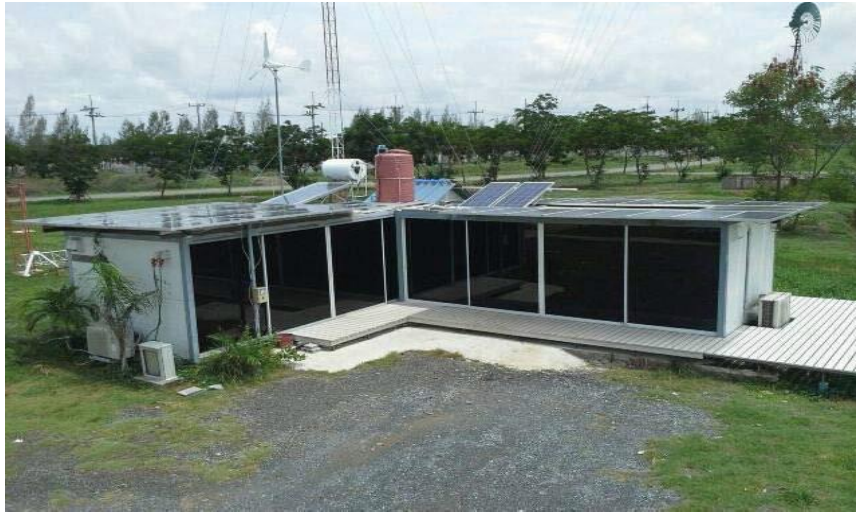
Figure 1 Solar home at rural electrification learning center, King Mongkut's University of Technology Thonburi (Bangkuntien)
