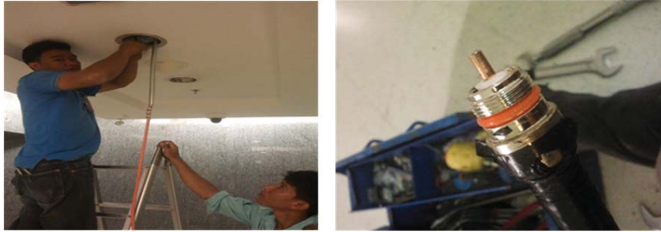
Figure 8: Antenna install to the ceiling and too long of inner conductor, one of high PIM value problems.
